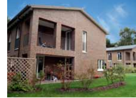
Building and maintaining these family houses at an SOS Children's Village near Hamburg is supported by Dr. Oetker.
